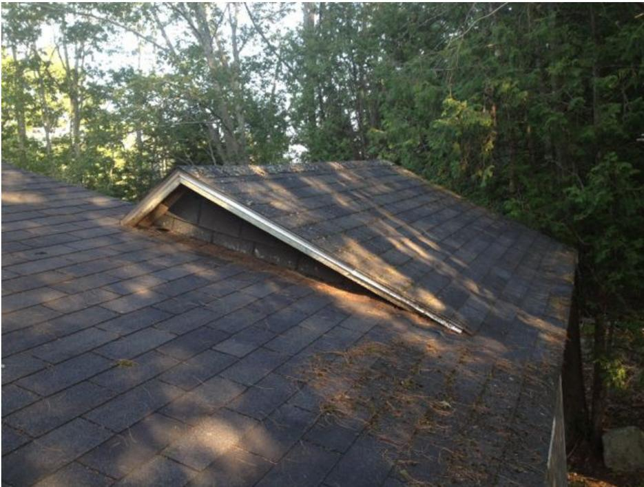
The way the roof is set up now, there's a gap as the two surfaces go down to meet, three courses up from the bottom. I would propose to remove the shingles immediately next to and under this overhanging gable, attach solid wood to bring the gable face out flush with the upper roof edge, re-shingle the lower surface with proper step flashing, and face the new vertical boarding with solid flashing tucked under the drip edge above. Trying to get everything watertight when it's recessed
