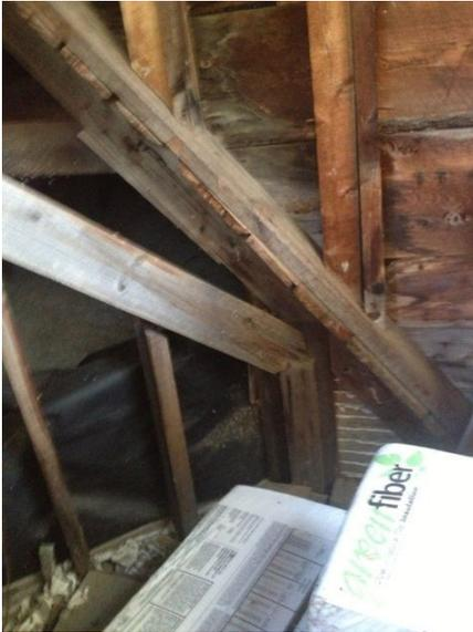
I saw no evidence of dripping on the top of the new cellulose insulation. This makes me think the water marks may be old, but I'm not certain. The way to know is to paint the area of the ceiling and see if the water marks re-appear.
